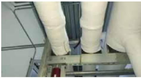
Cold water flow meter detector
